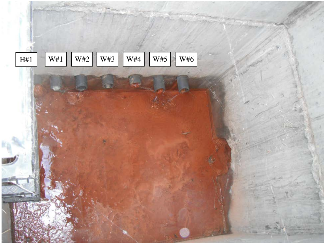
Figure 2, Photograph of Outlet Pipes Taken on 6/20/14
