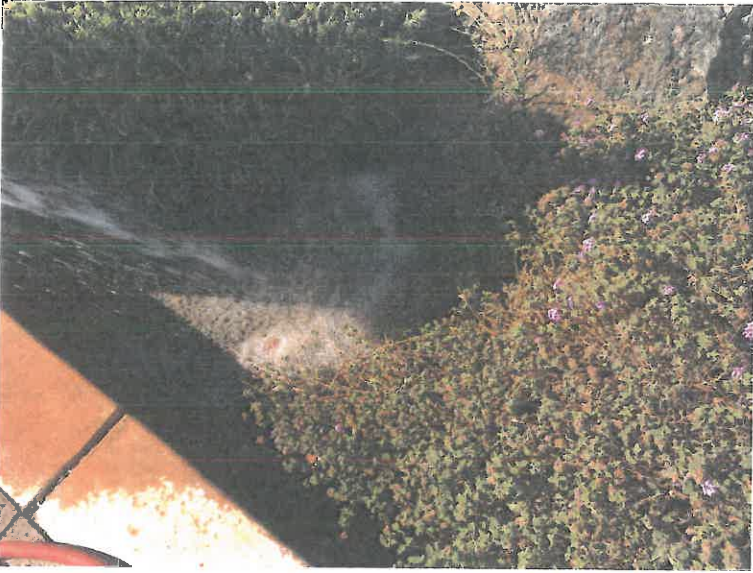
Oakhurst Water Feature Planter # 2 Water test
