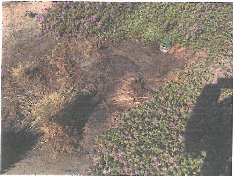
Oakhurst Water Feature Planter # 1 water test
