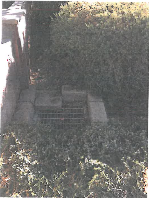
Clayton Community Park DI planter # 2 | reset 6 inch dam
