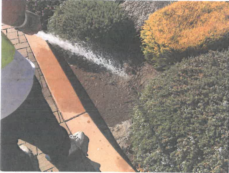
Oakhurst Water Feature Planter # 3 water test
