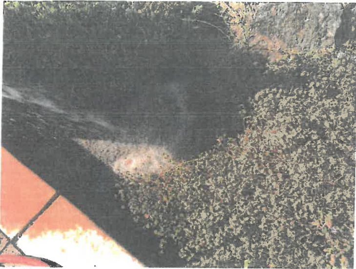
Oakhurst Water Feature Planter # 2 Water test
