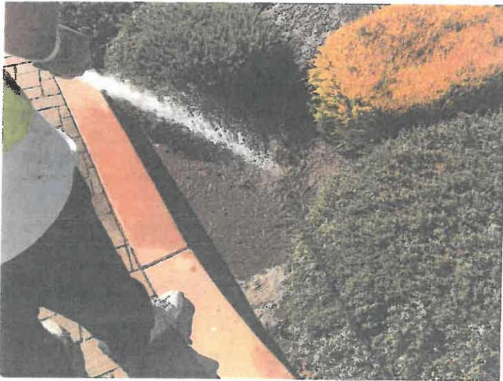
Oakhurst Water Feature Planter # 3 water test
