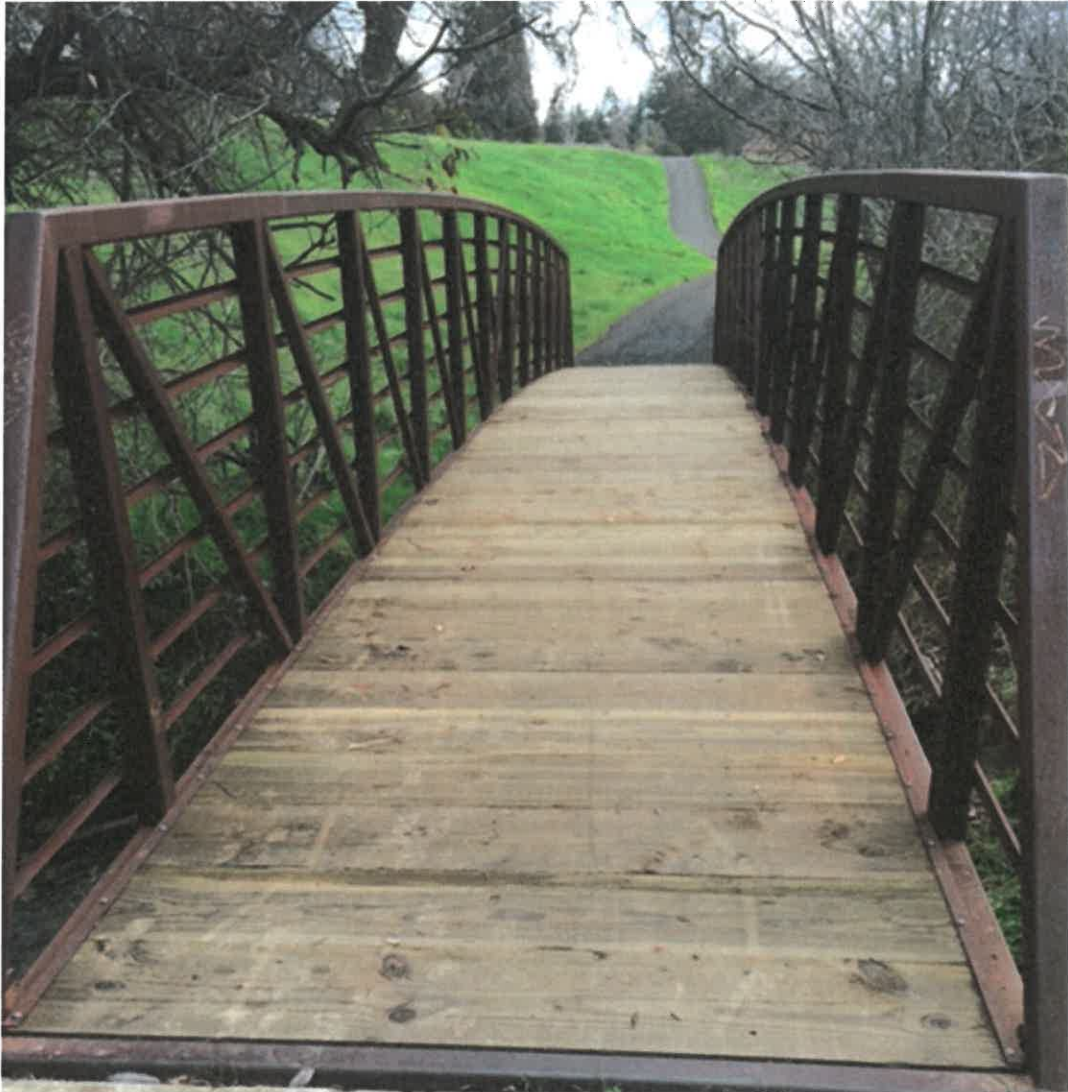
After replacement of wood deck
