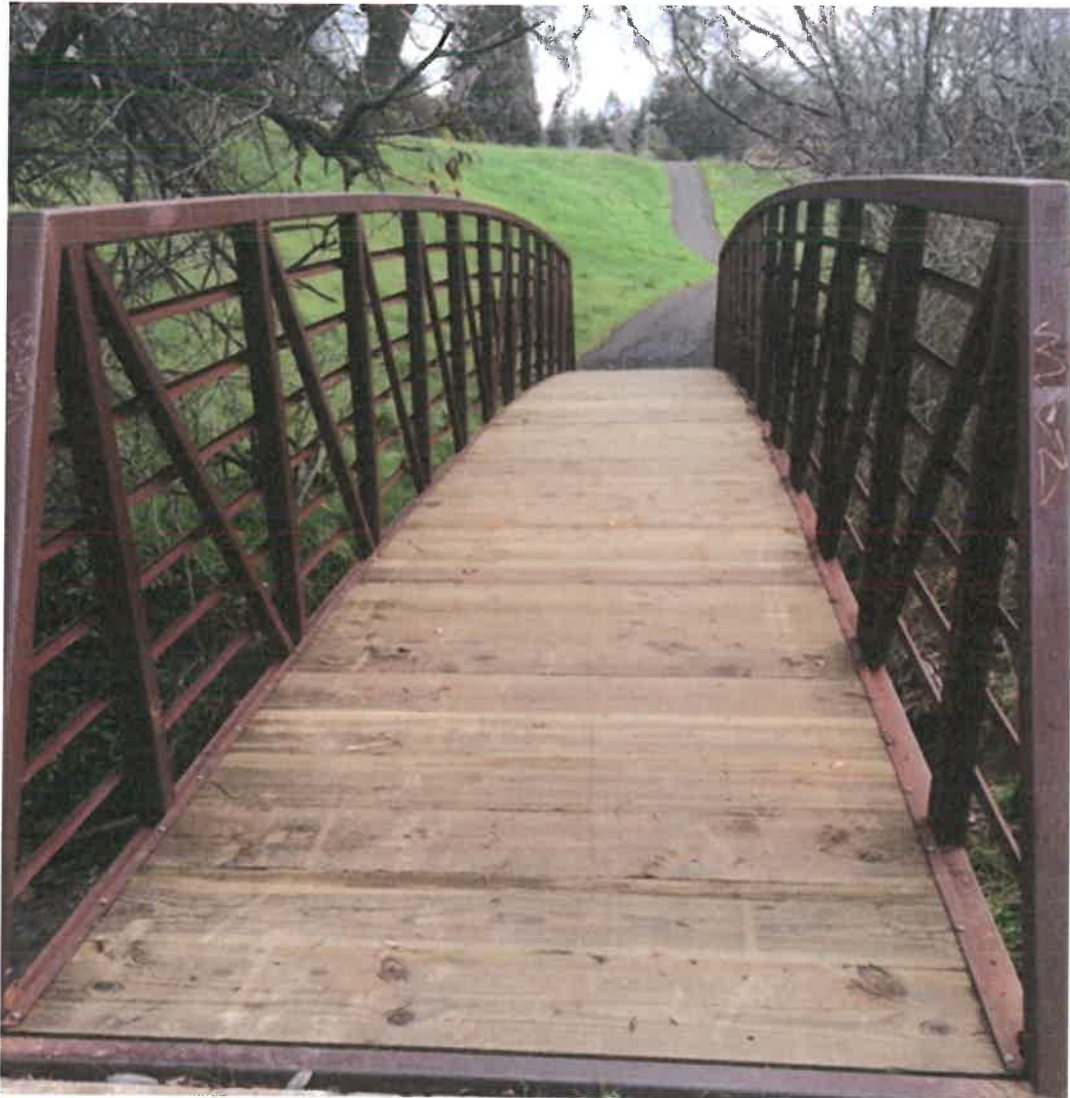
After replacement of wood deck
