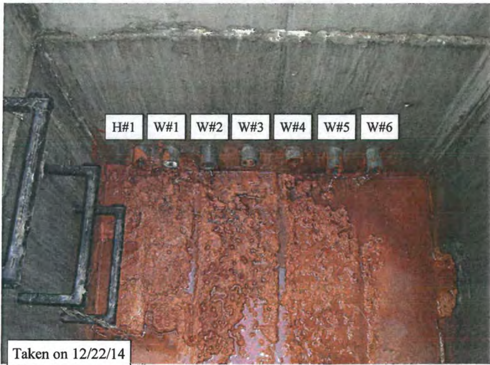
Figure 2, Photograph of Outlet Pipes
