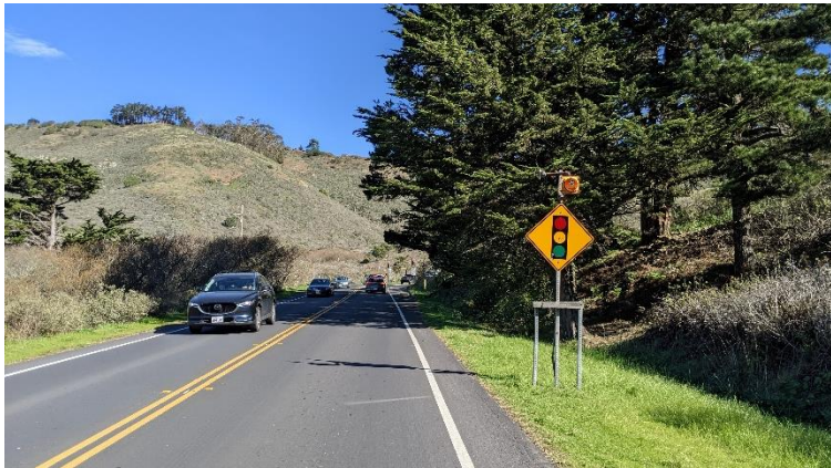
Figure 3 Example of Flashing Beacons as Advance Warning
