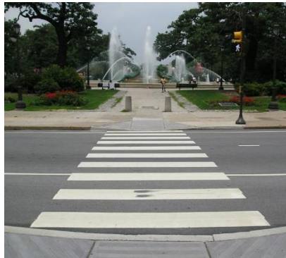
Figure 11 Example of a High Visibility Pedestrian Crossing
