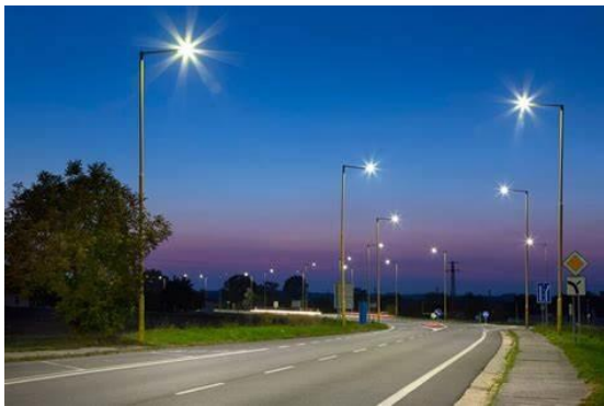
Figure 14 Example of Roadway Segment Lighting
