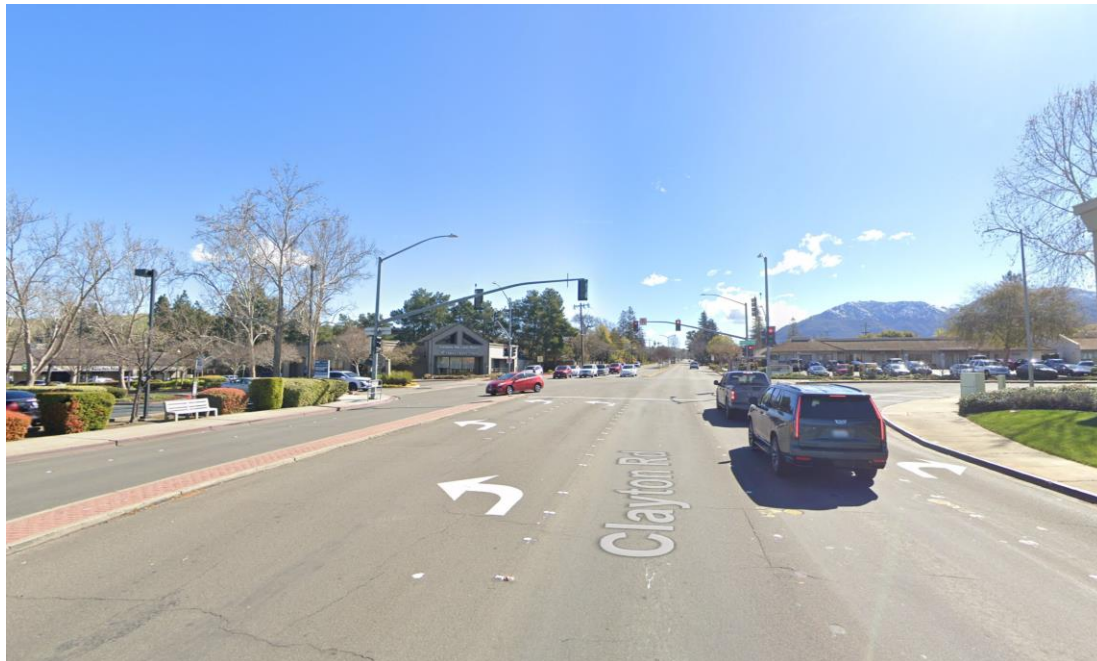
Figure 2 Example of Existing Left Turn Lane - Clayton Road, City of Clayton
