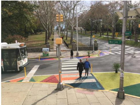
Figure 12 Example of a Curb Extensions and Advanced Stop Bar
