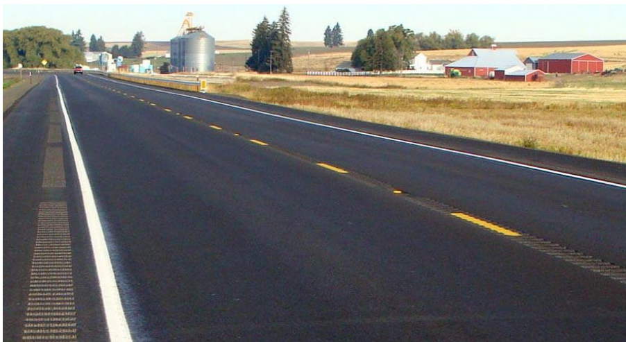
Figure 18 Example of Edgeline Rumble Strips
